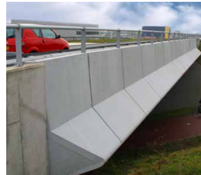
Fly-over panels - Amersfoort, The Netherlands - Be Concrete
